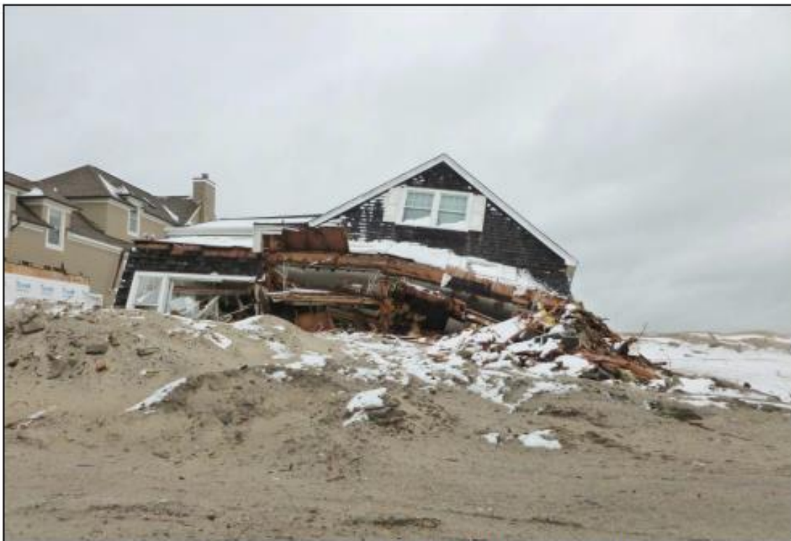
Image #2: The above example photo illustrates pancaking.
