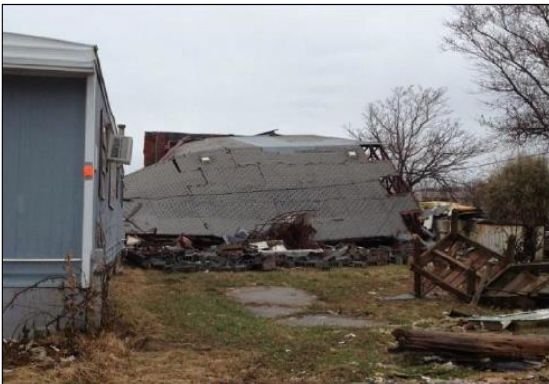
Image #5: The above example photo illustrates a building where the roof has collapsed.
