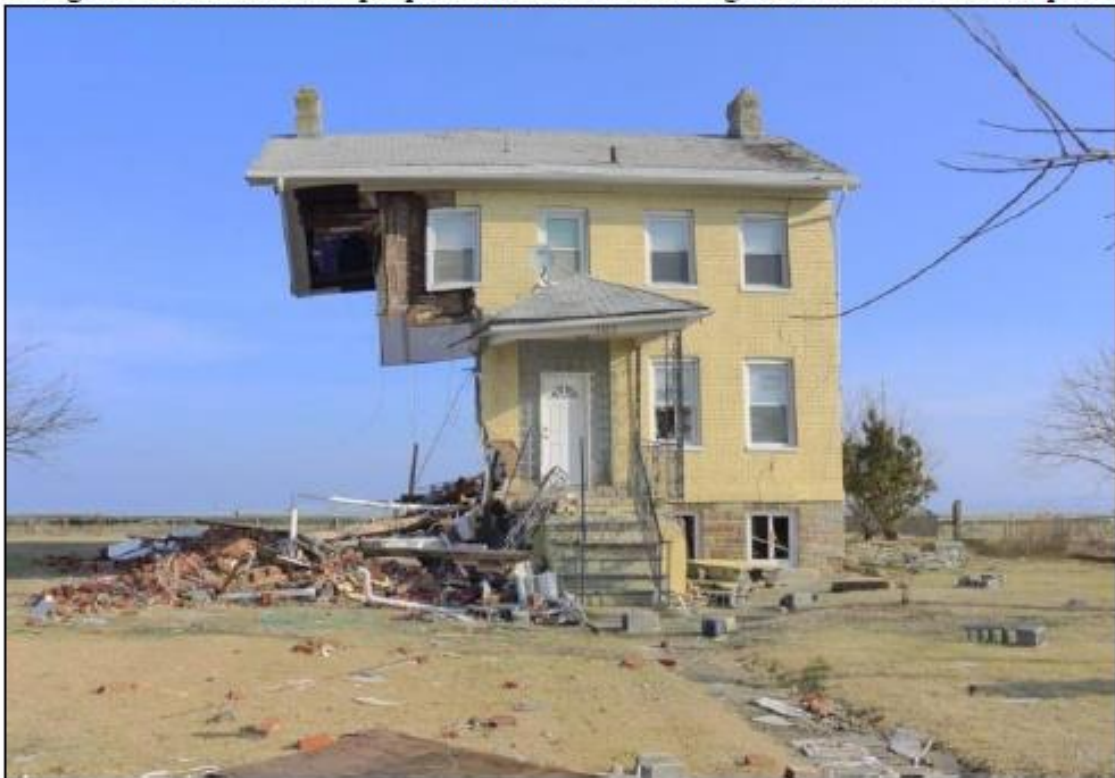
Image #6: The above example photo illustrates a building that is missing one or more complete elevations.
